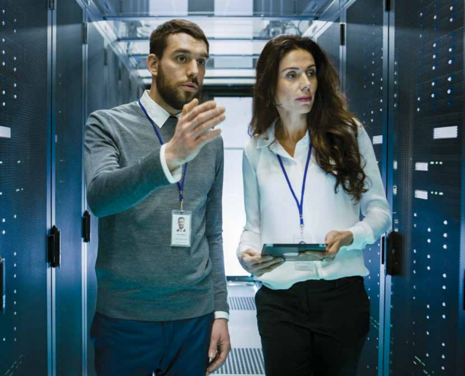
Protecting content production, storage and delivery of broadcast and multimedia services from cyber threats relies on both IT and operational technology (OT)
