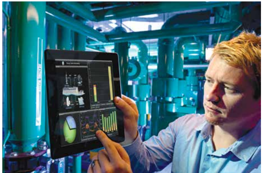
Human machine interfaces are widespread across transmission and distribution networks (Photo: CSIRO Wikimedia Commons)
